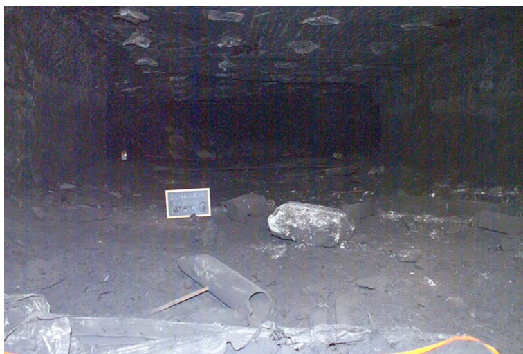
Photo 4. Location: Seal #3 (Courtesy of MSHA)
