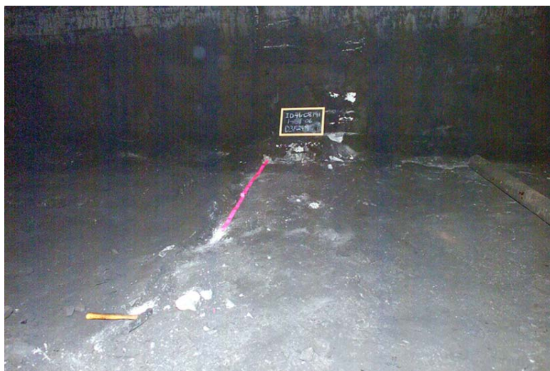
Photo 7. Location: Seal #6 (Courtesy of MSHA)
