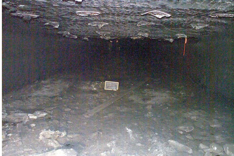
Photo 11. Location: Seal #10 (Courtesy of MSHA)
