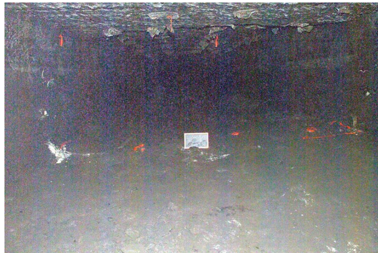
Photo 6. Location: Seal #5 (Courtesy of MSHA)
