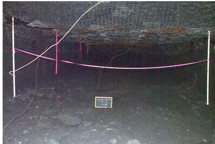
Photo 9. Location: Seal #8 (Courtesy of MSHA)
